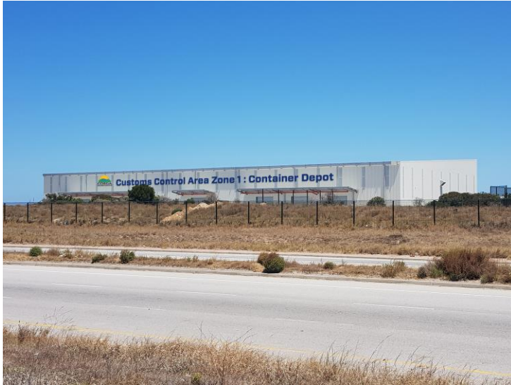
Coega Customs Control Area 3600 m2 Warehouse
