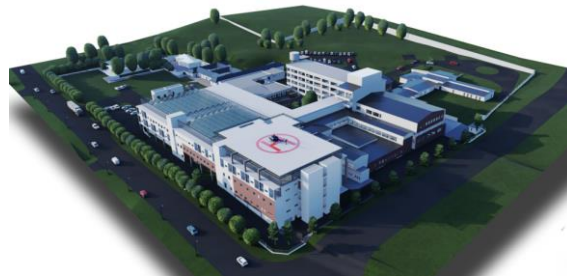
Artist impression of the Dihlabeng Regional Hospital, located on the N5 national road in Bethlehem in the Free State.
