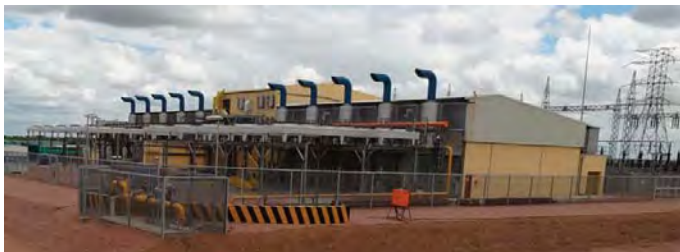
Financing, construction, erection, commissioning, operation and maintenance of a 40MW natural gas fired power plant and Project Facilities at Chokwe, Gaza Province, Mozambique.
