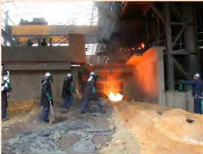
Furnace at SA chrome facility
