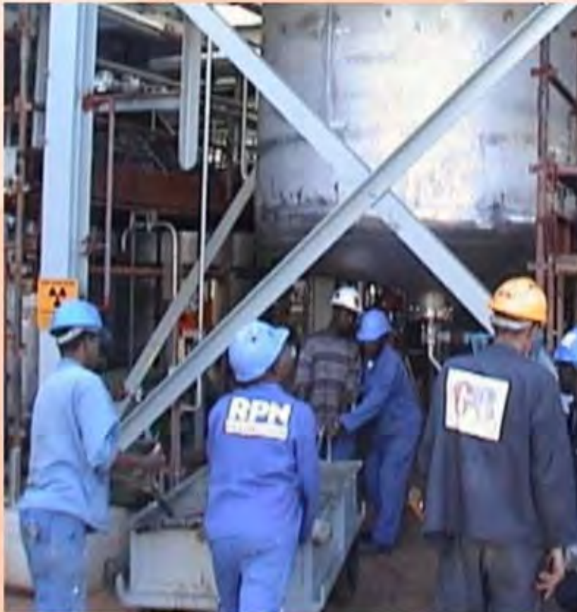
Installation of a cooling crystalliser on SA bioproduct
