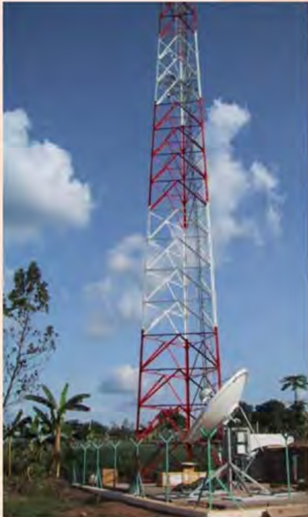
Towers - Wireless Communication Equipment made in South Africa for export sales
