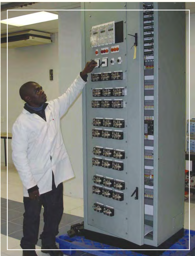
A Test Technician at the ALSTOM Protection & Control site performing functional checks on a Bus Zone Protection Scheme for export to Sudan.
