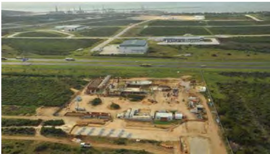
Coega SEZ shows construction activity, with the Port of Ngqura in the background
