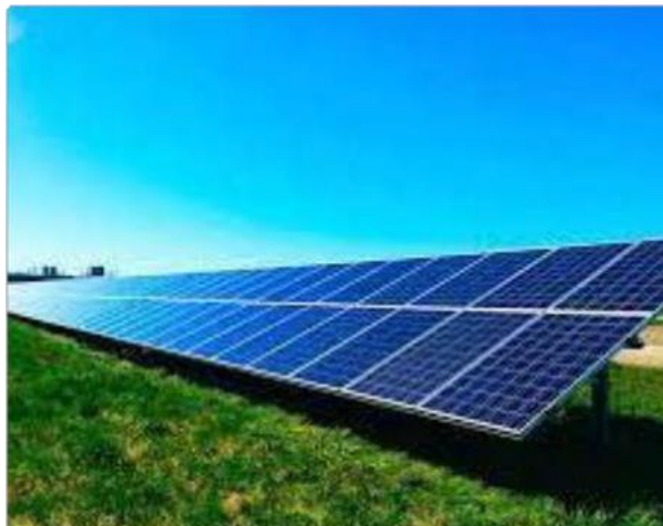
Construction of a solar energy plant.
